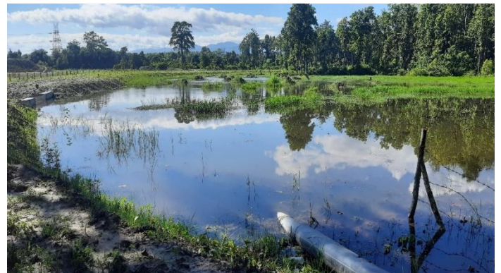
Work after photograph:
