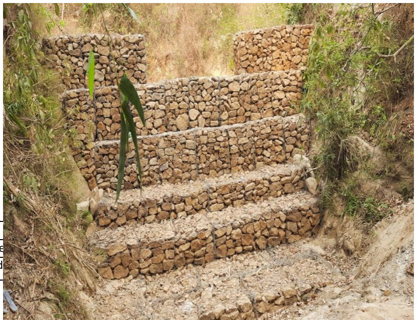
Work after photograph:
