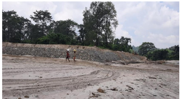
Work after photograph:
