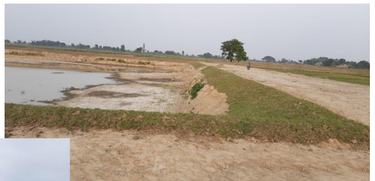
Work after photograph:
