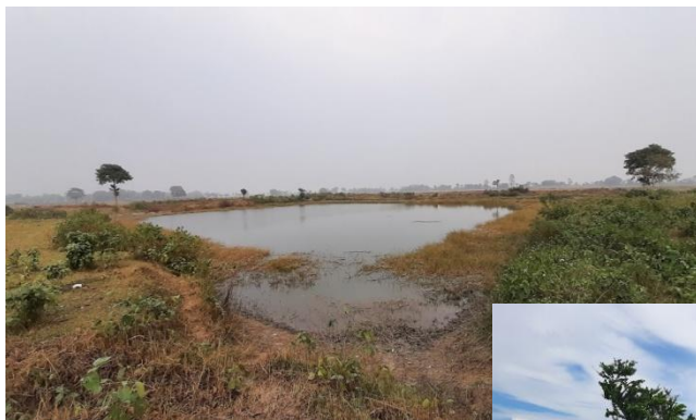
Work before photograph:
