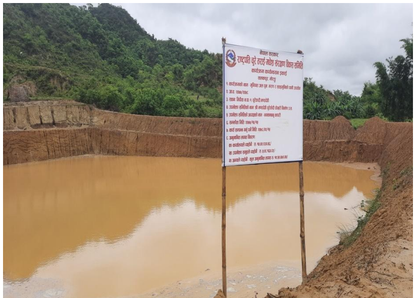
Work after photograph:
