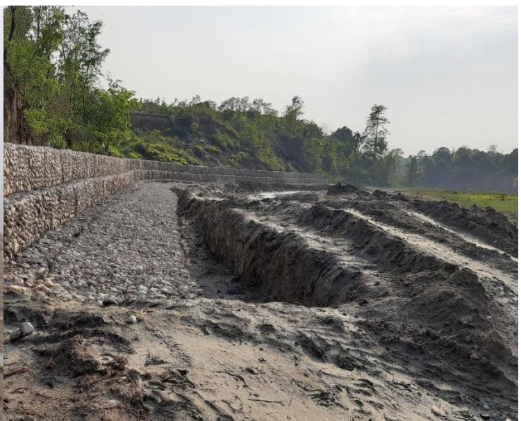
Work after photograph:
