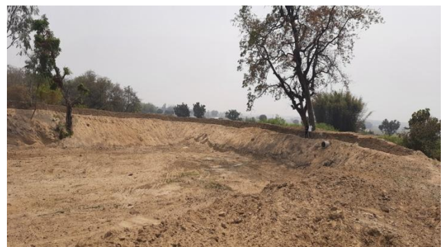
Work after photograph:
