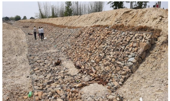
Work after photograph:
