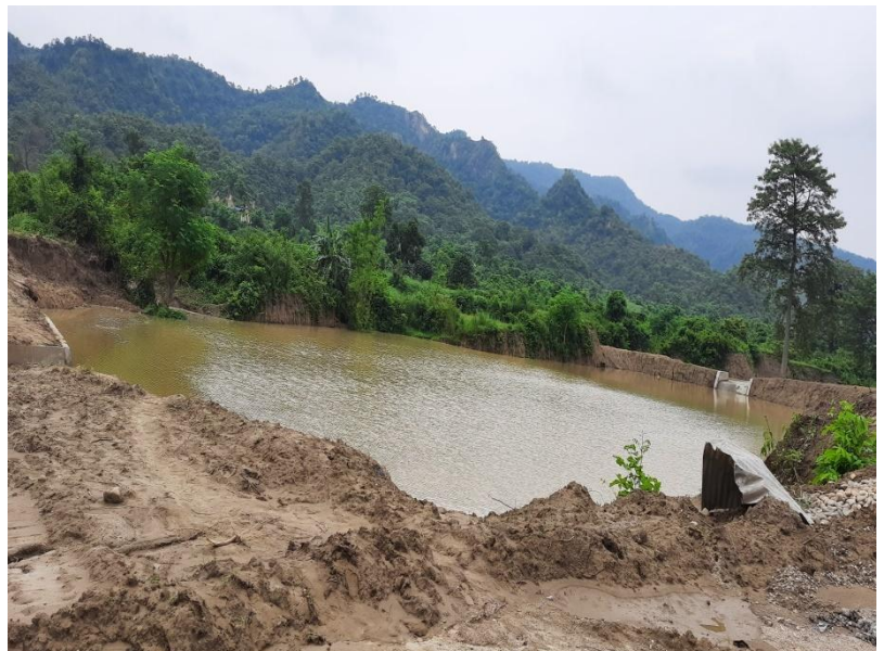
Work after photograph:
