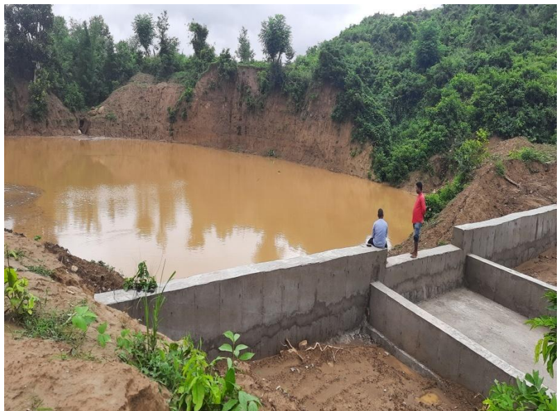
Work after photograph:
