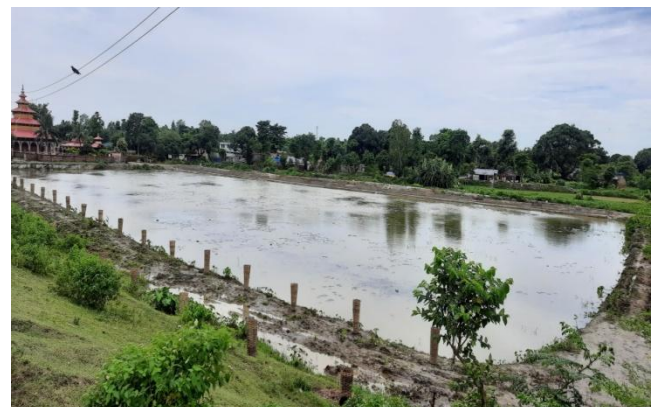
Work after photograph:
