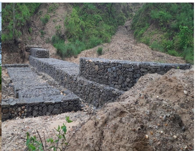
Work after photograph:
