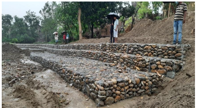
Work after photograph:
