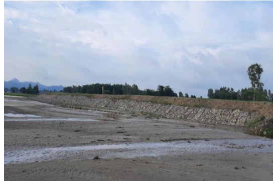
Work after photograph:
