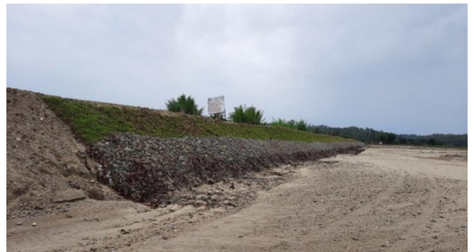
Work after photograph:
