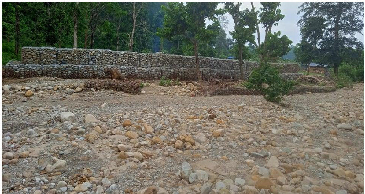
After Work Completion
