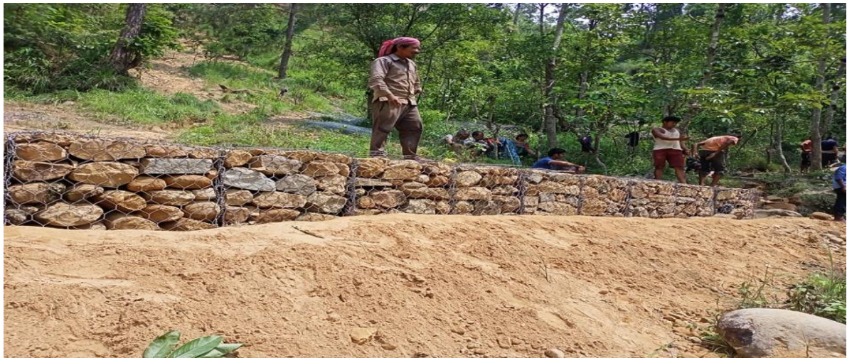
After Work Completion
