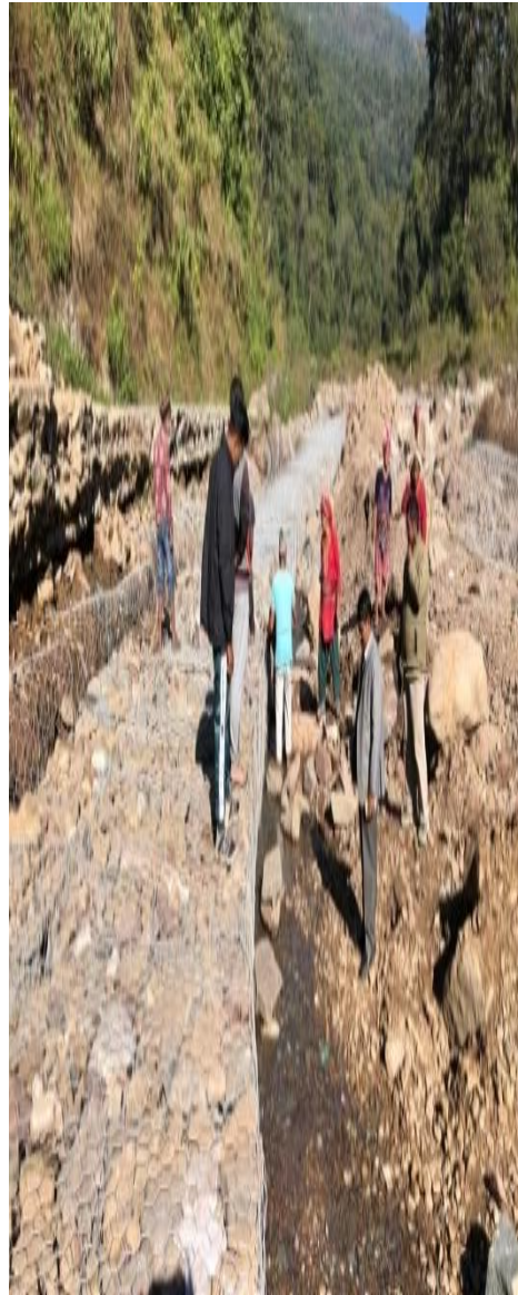
Work on progress
