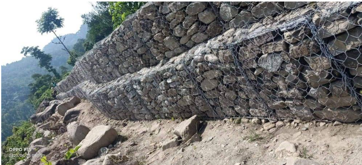
After Work completion
