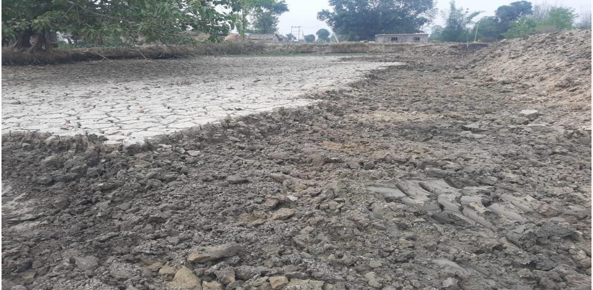
During the Work
