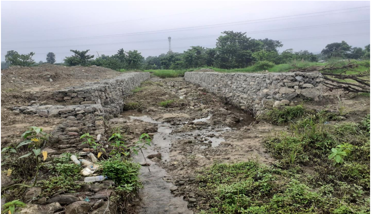
After Work Completion
