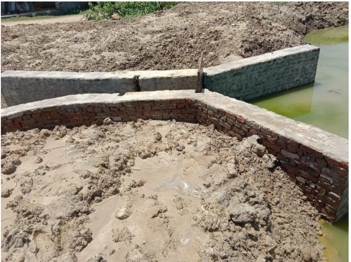
After work completion
