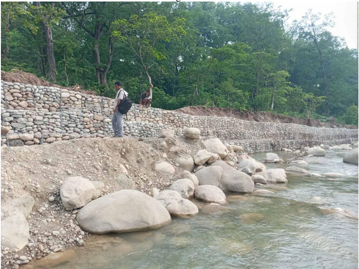
After Work Completion
