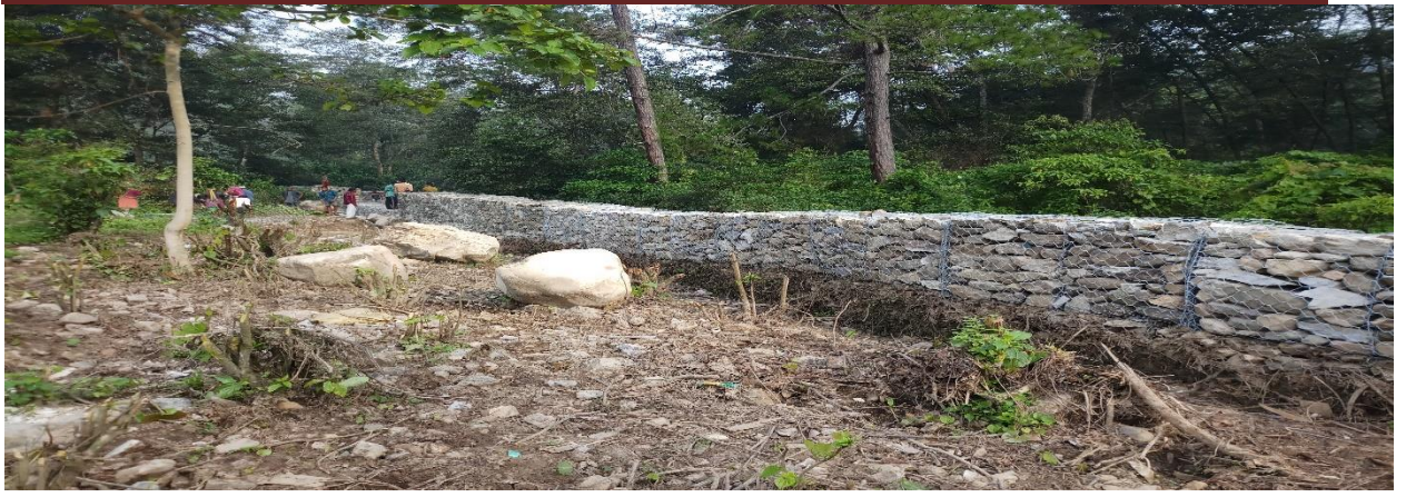
After Work Completion
