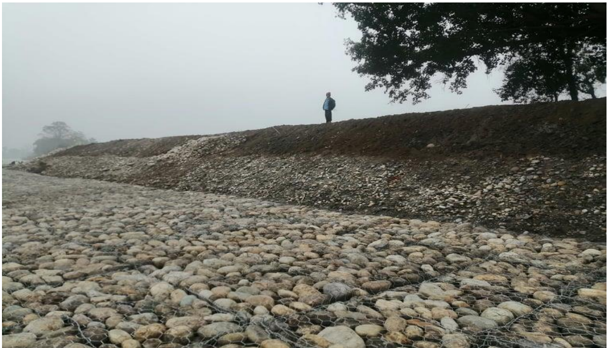
After Work Completion
