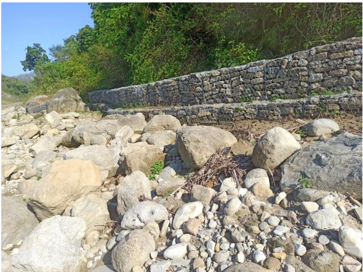
After Work Completion
