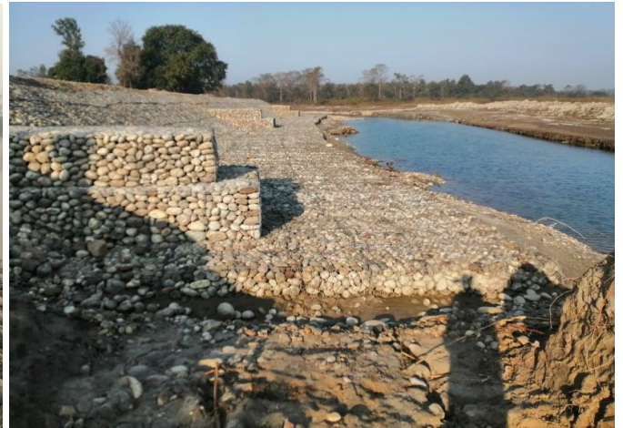
After completion of work
