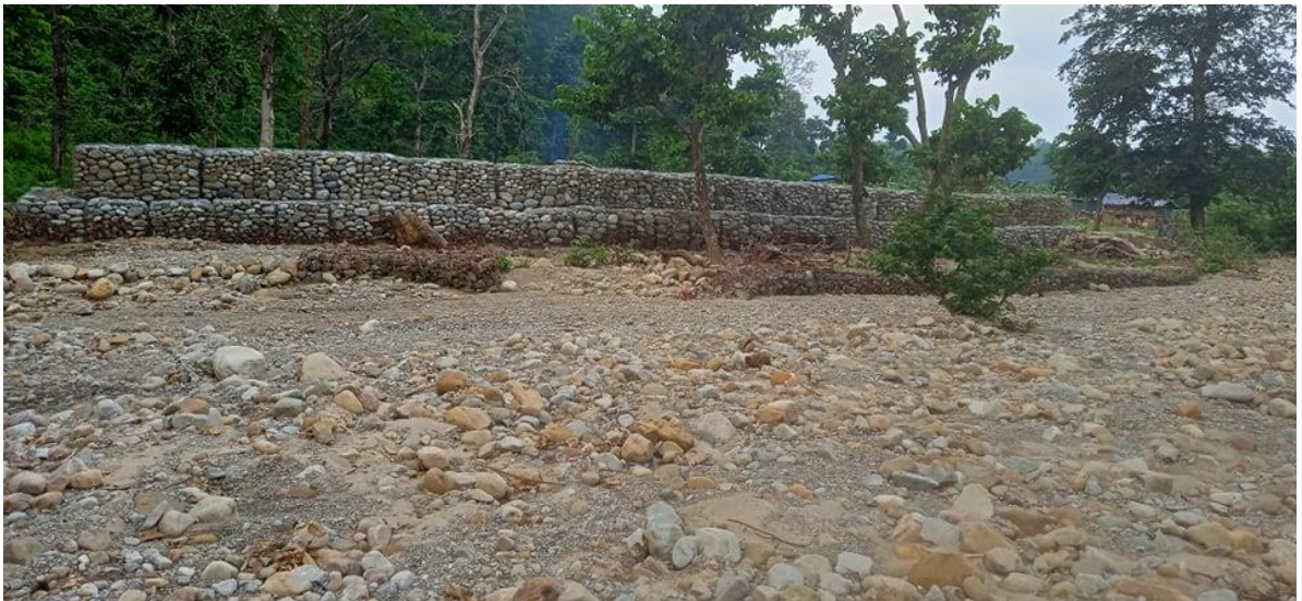
After Work Completion
