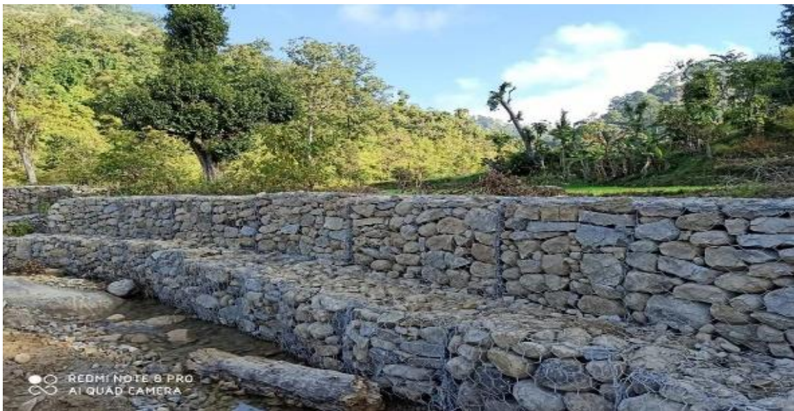
After Work Completion
