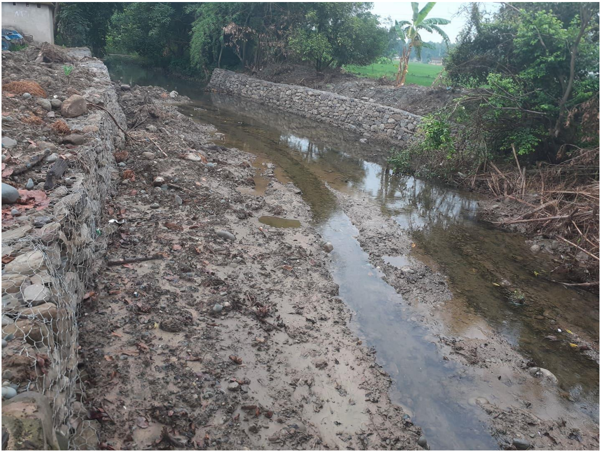
After Work Completion
