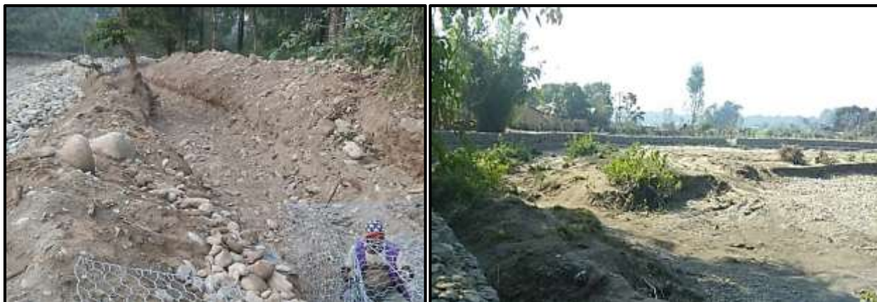
After work completion
