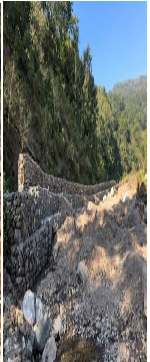
After work completion
