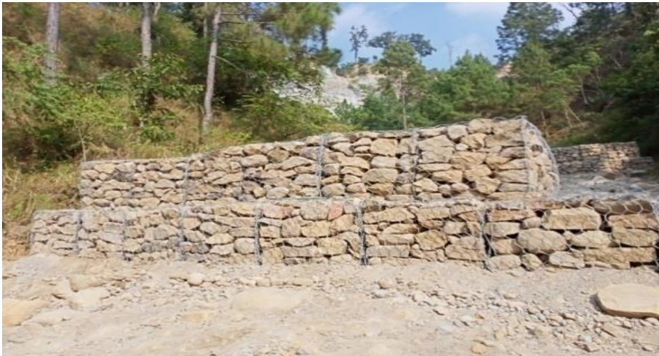
After Work Completion
