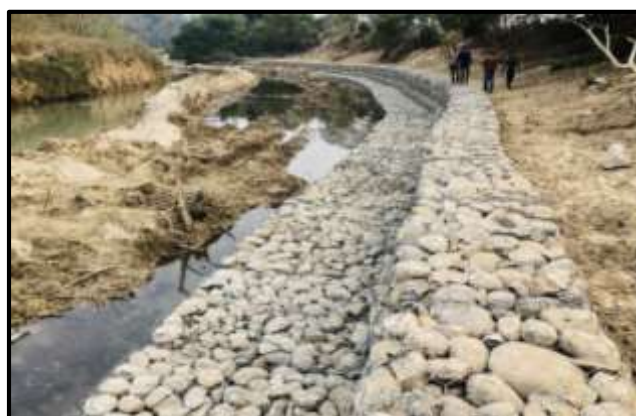
After completion of the project
