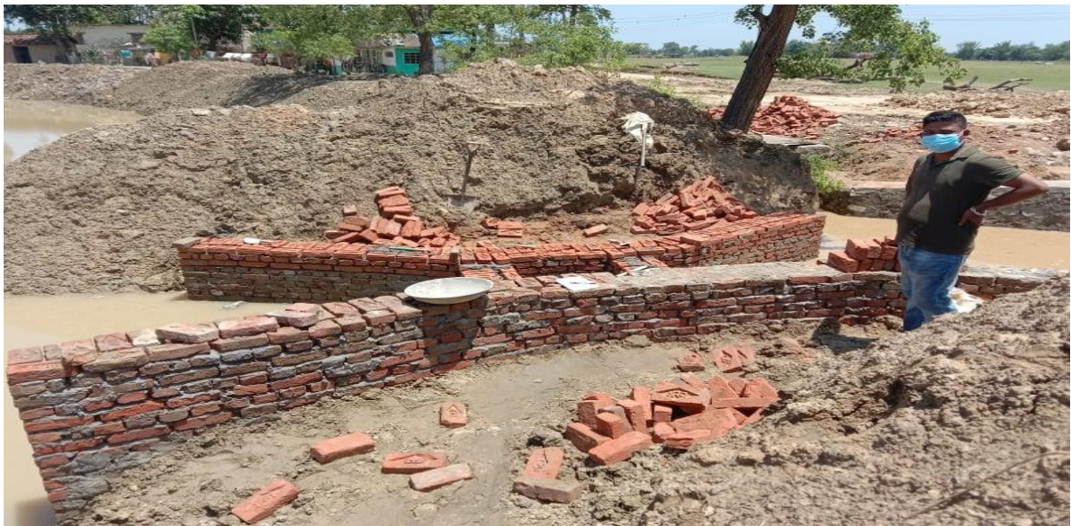
After work Completion
