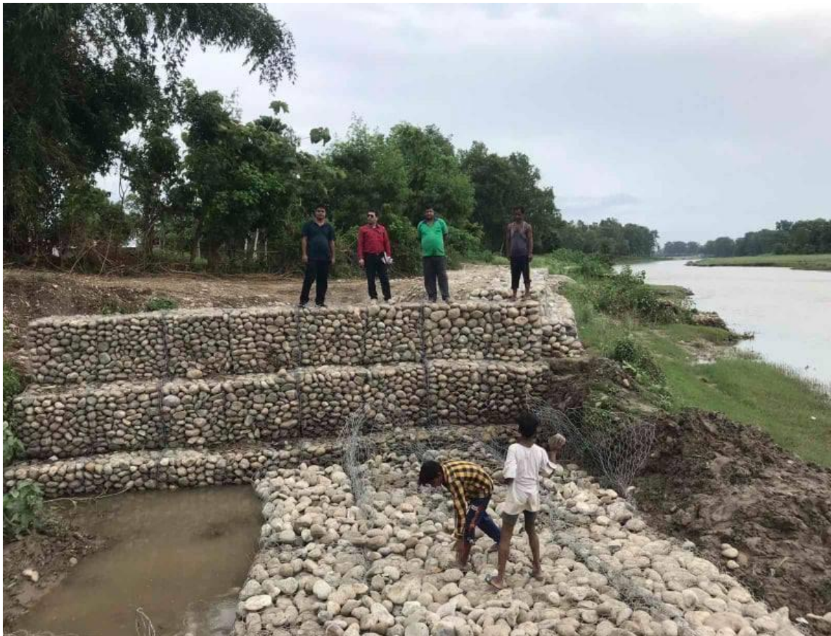
After Work Completion
