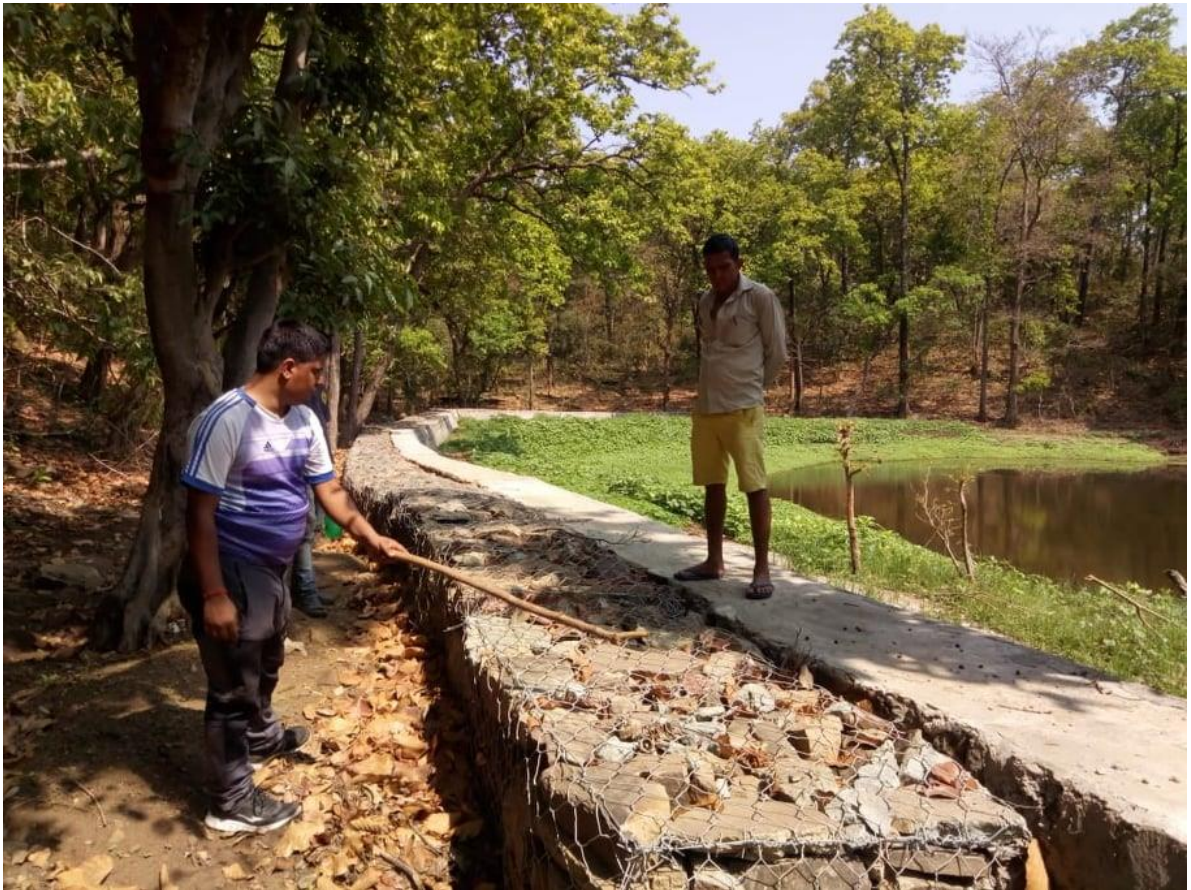
After Work Completion
