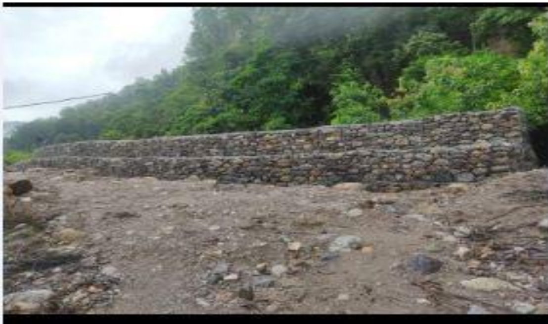
After Work Completion
