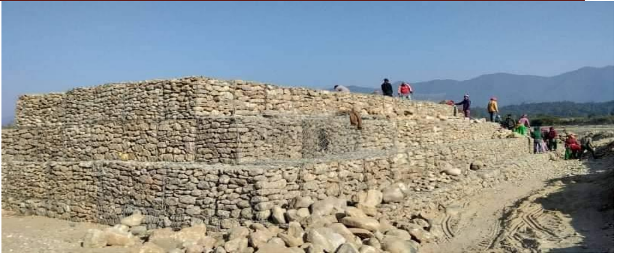
After Work Completion
