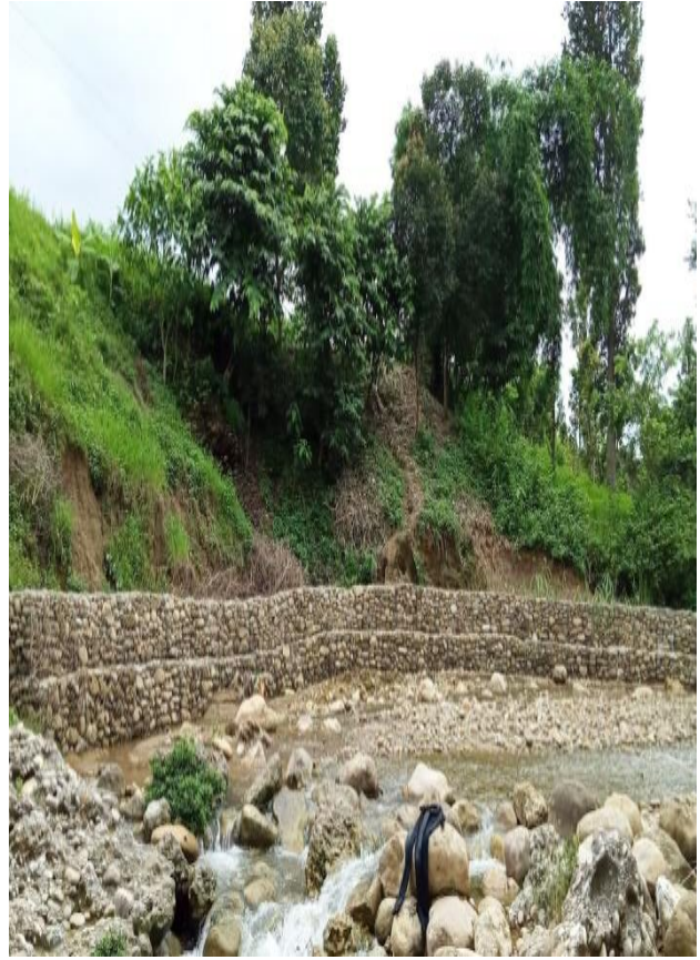
After work completion
