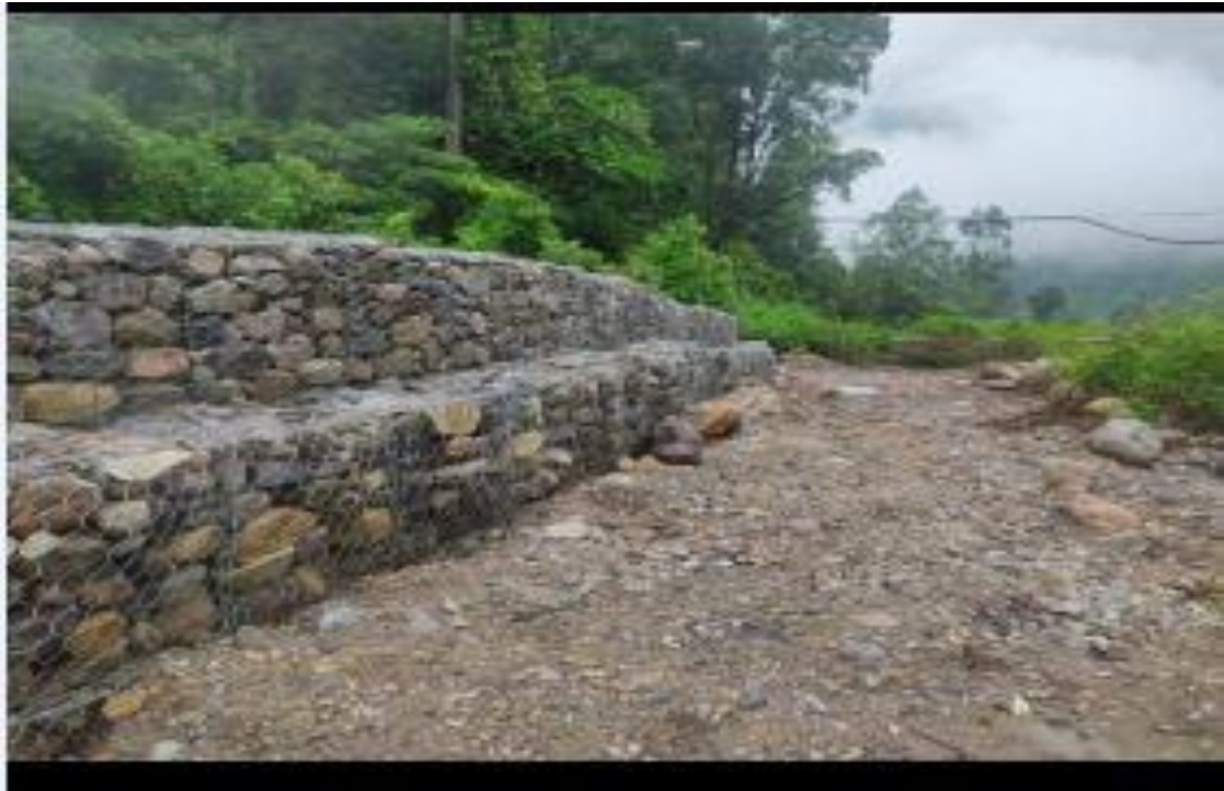
After Work Completion
